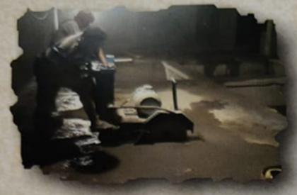
RCC SLAB CUTTING WITH CUTTER MACHINE
