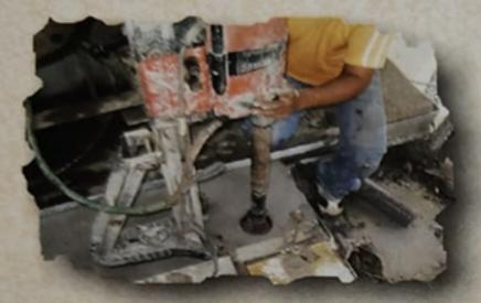
CORE DRILLING IN RCC FOUNDATION UPTO 1.5 MTRS. DEPTH
