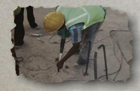
FILLING CHEMICAL IN HOLES FOR COMPLETING REBARING WORK
